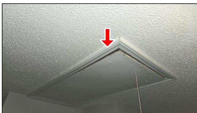
F. Item 5(Picture) pull down attic stairs
