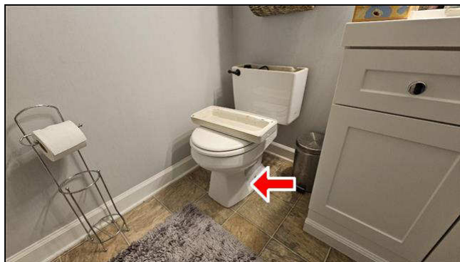
A. Item 8(Picture) upstairs hall bathroom
