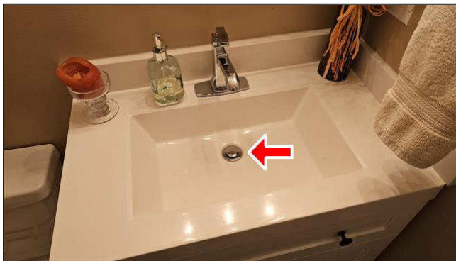
A. Item 7(Picture) downstairs bathroom sink
