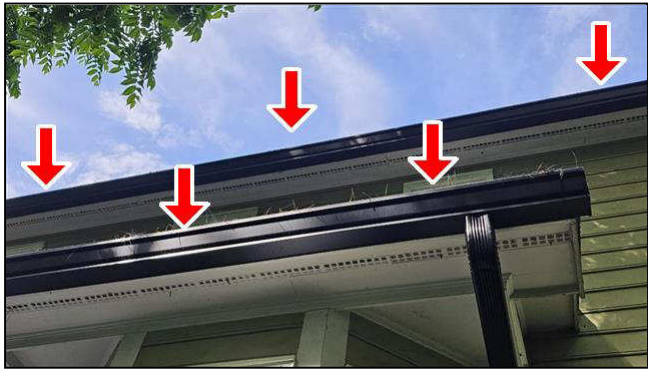
D. Item 2(Picture) rear roof
