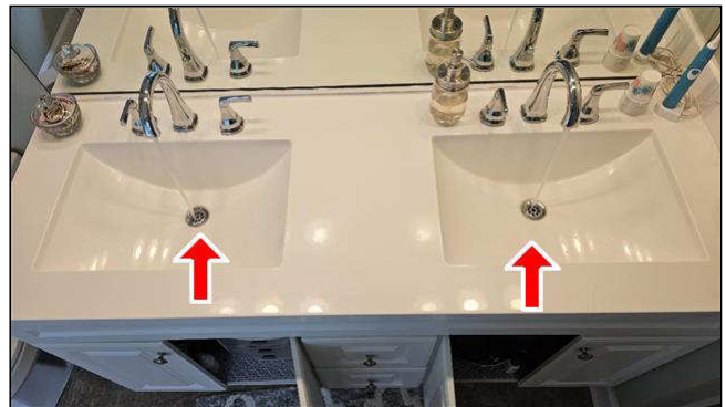
A. Item 6(Picture) primary bathroom sinks
