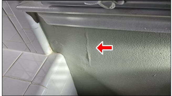
B. Item 4(Picture) primary bathroom front window
