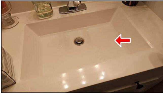
A. Item 4(Picture) downstairs bathroom sink
