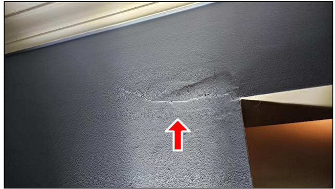
B. Item 2(Picture) front dining room entry
