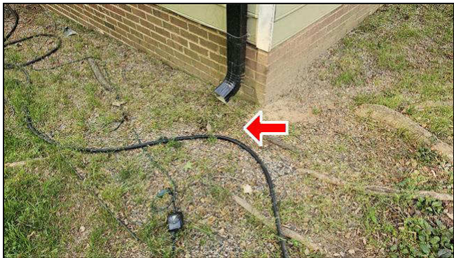
D. Item 1(Picture) rear left corner
