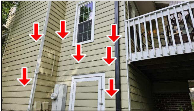
A. Item 3(Picture) right rear wall
