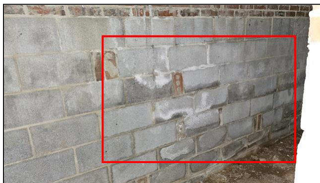
A. Item 1(Picture) front wall under porch
