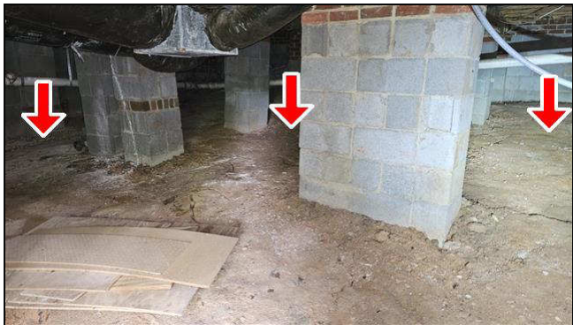
C. Item 1(Picture) throughout crawlspace
