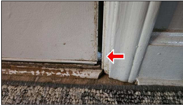
B. Item 1(Picture) door to garage
