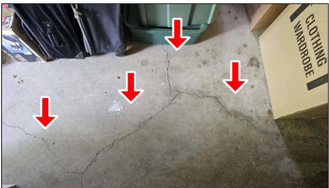
C. Item 2(Picture) garage
