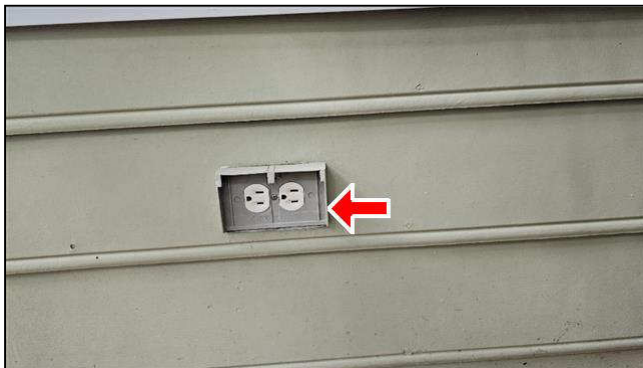
D. Item 6(Picture) rear deck
