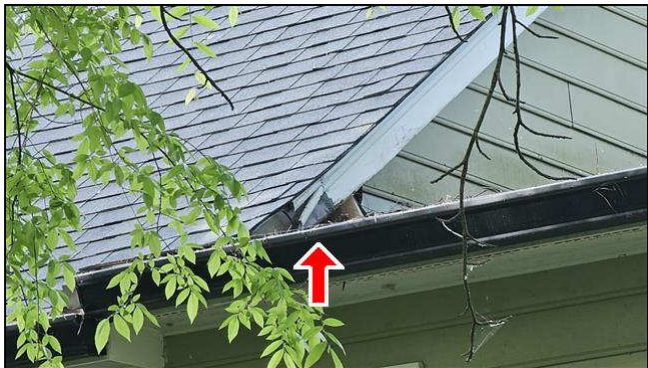
F. Item 1(Picture) rear roof
