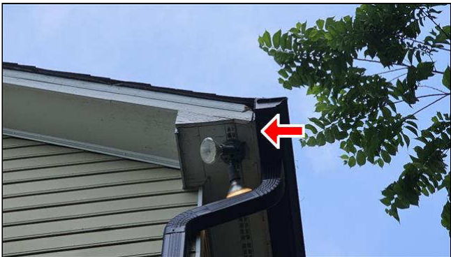
F. Item 2(Picture) rear right corner
