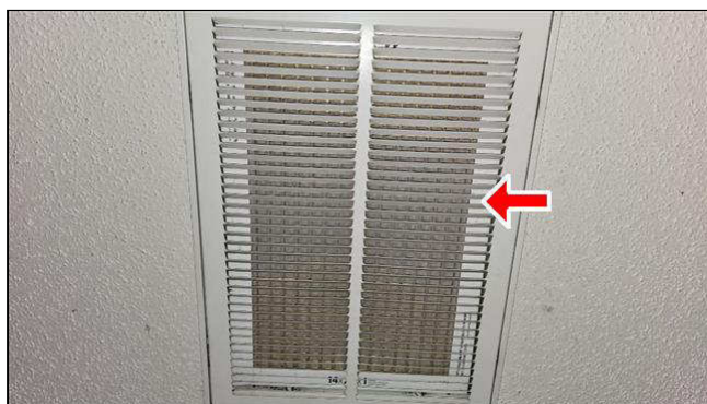
D. Item 1(Picture) upstairs hall
