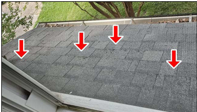
A. Item 2(Picture) front porch roof
