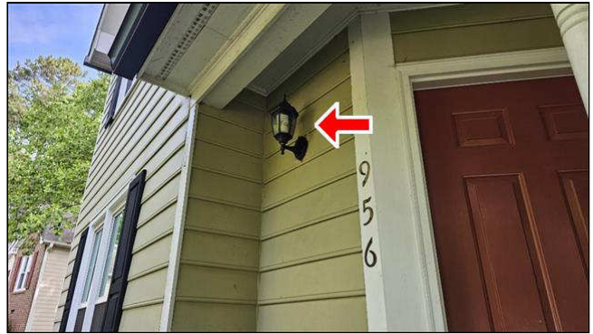
D. Item 4(Picture) front porch
