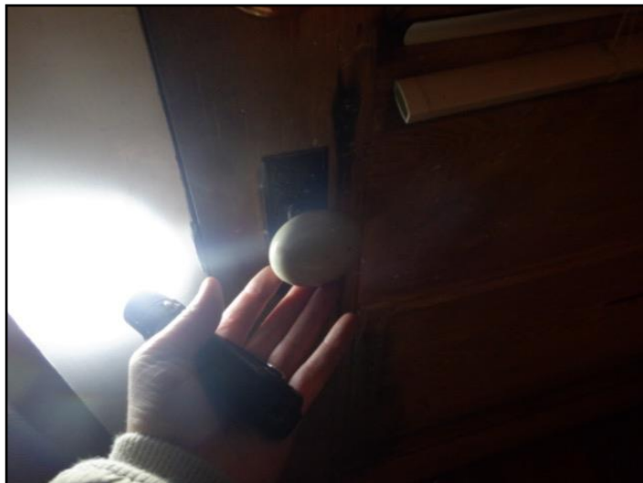
General door issues
