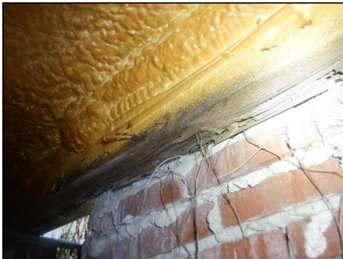
Rot or insect damage
