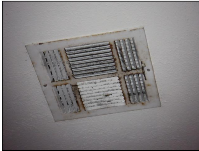
Possible mold or microbial growth
