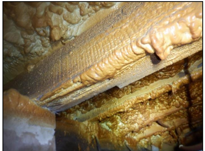
Rot or insect damage
