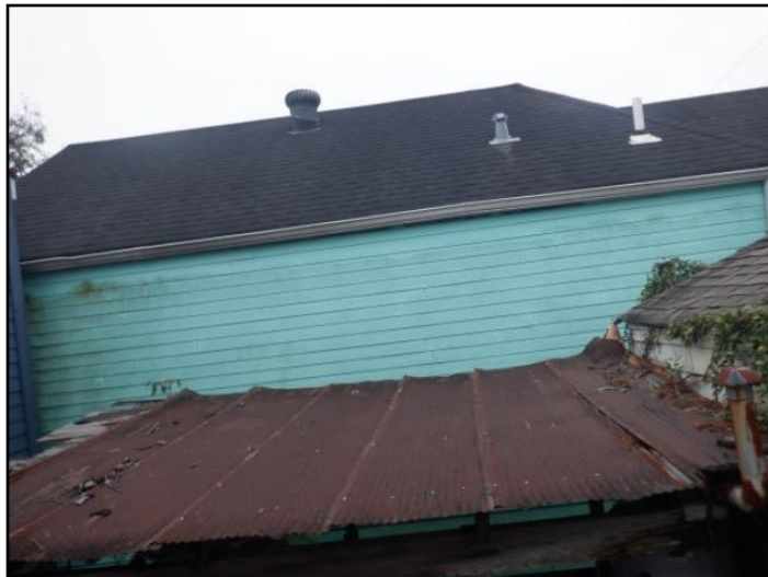
General View of the Roof System
