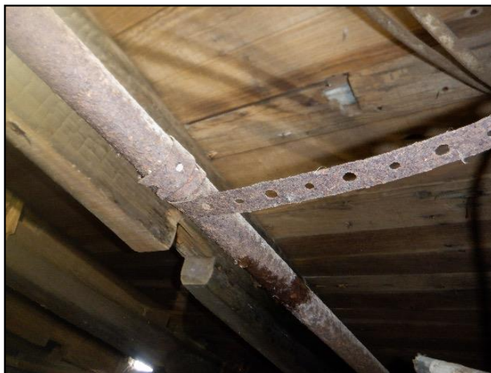
Inadequate support
