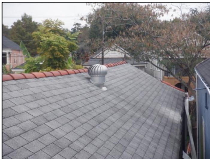
General View of the Roof System
