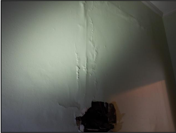
Water damage
