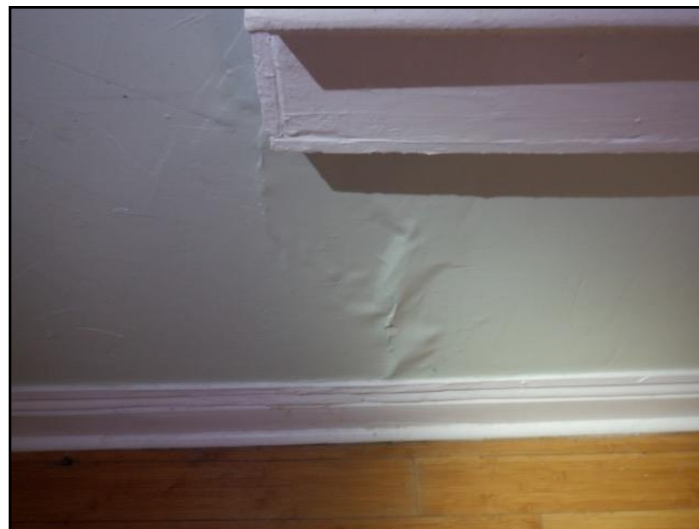
Water damage
