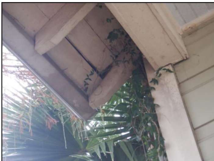
Rot/insect damage
