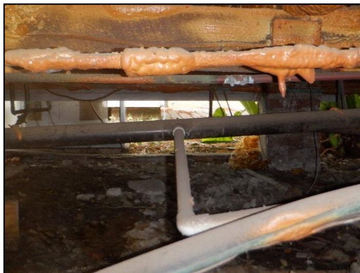
Reverse/improper slope
