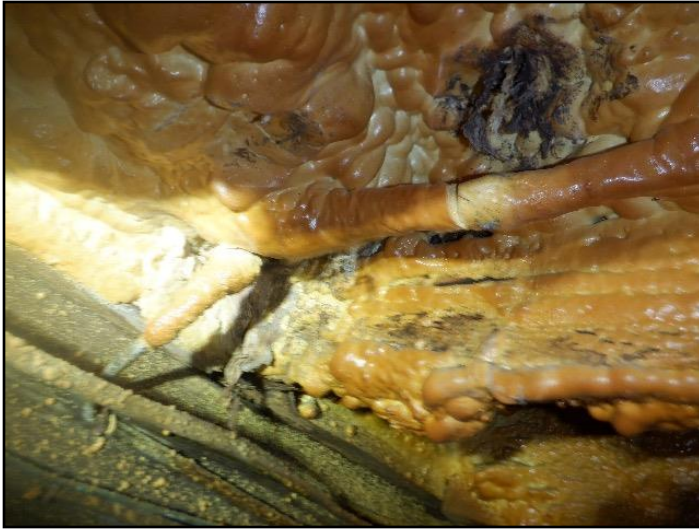
Rot and/or insect damage
