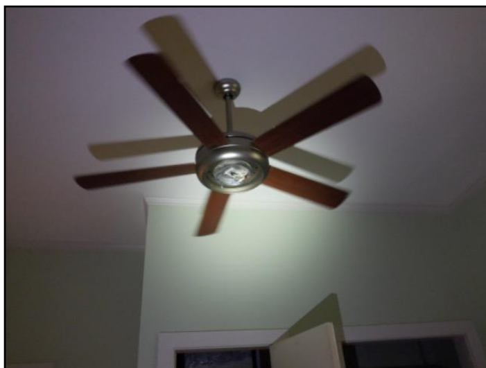
Trim kit or globe is loose or missing
