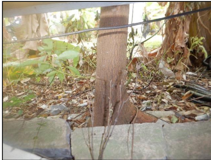
Large trees close to building
