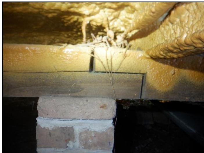
Improper splicing
