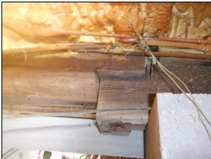
Improper splicing
