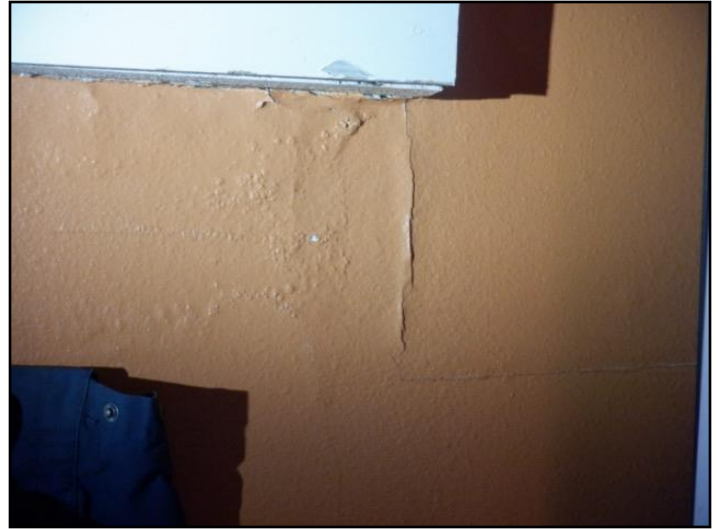
Water damage
