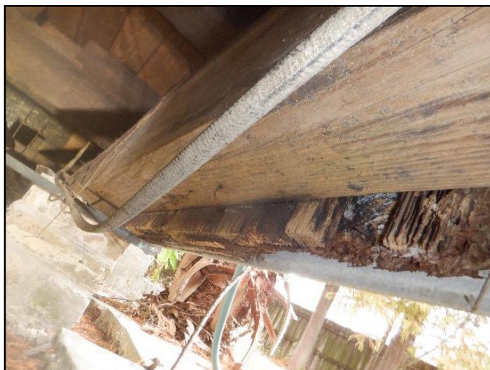
Rot or insect damage
