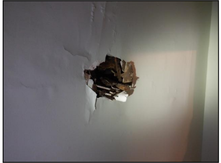
Water damage
