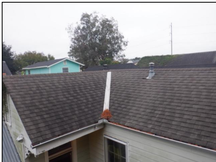
General View of the Roof System
