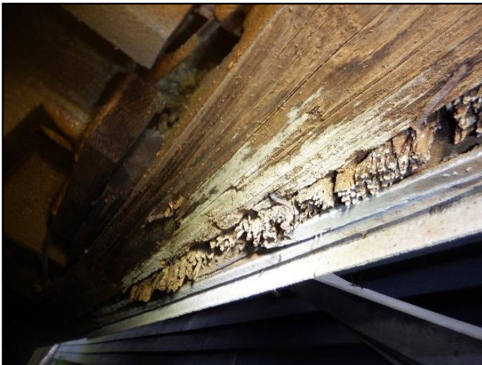
Rot or insect damage
