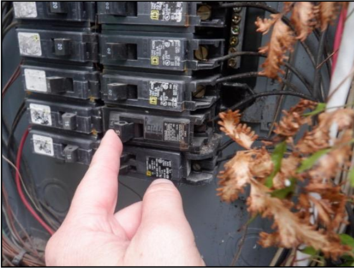
Undersized breakers may cause frequent...
