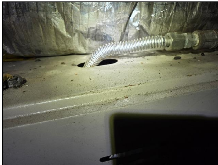
Passes through an appliance housing
