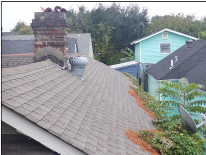
General View of the Roof System
