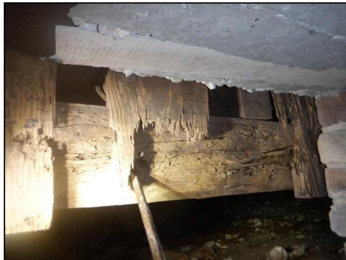
Rot or insect damage
