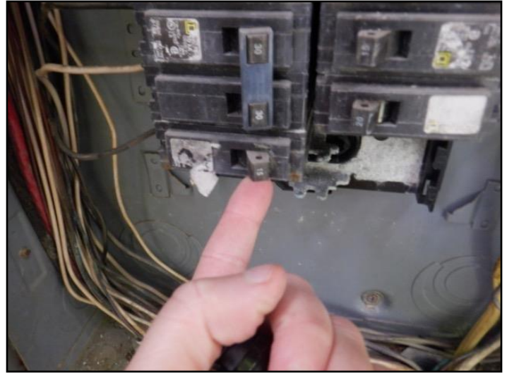
Undersized breakers may cause frequent...
