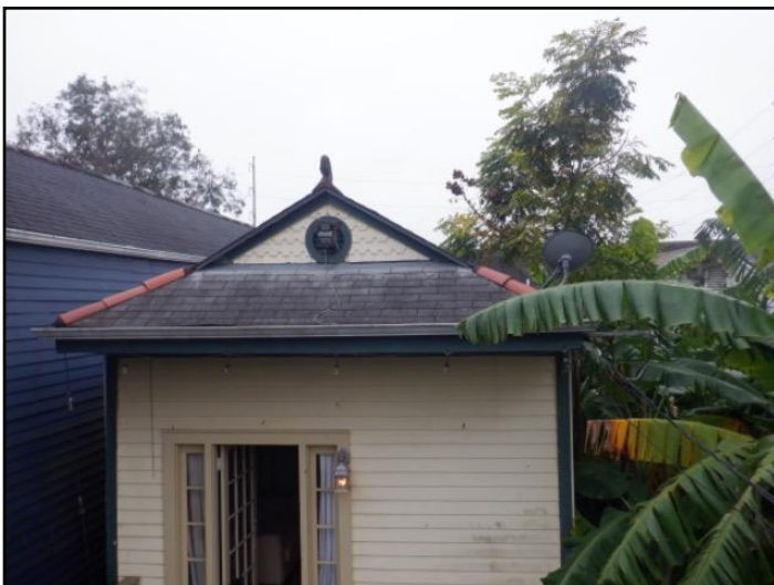
General View of the Roof System
