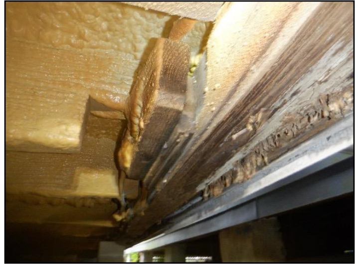
Rot or insect damage
