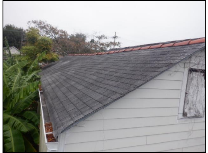
General View of the Roof System
