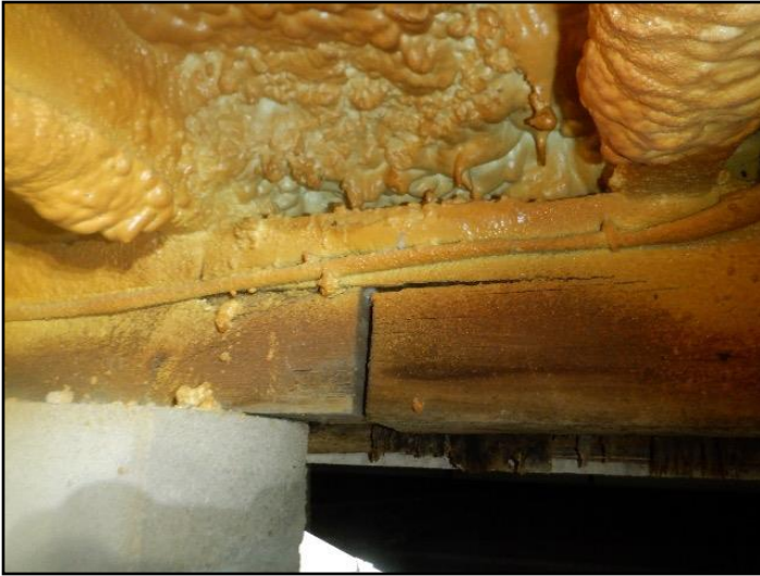
Improper splicing
