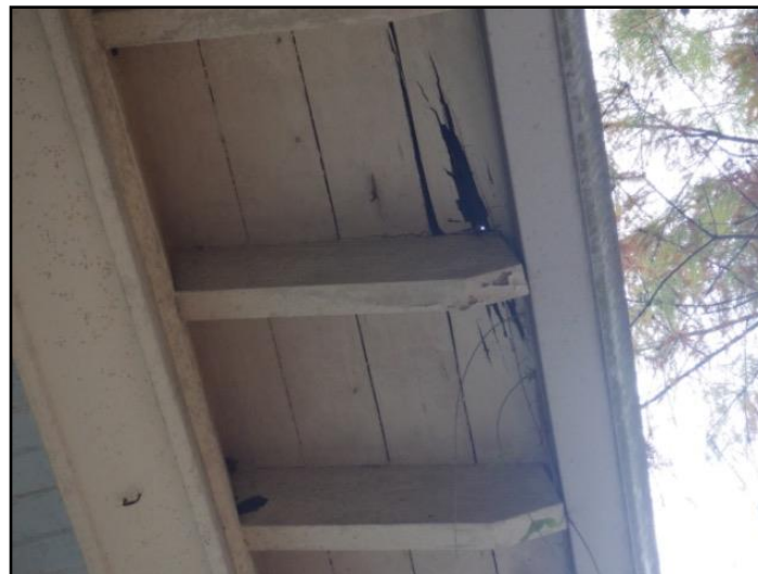
Rot or insect damage
