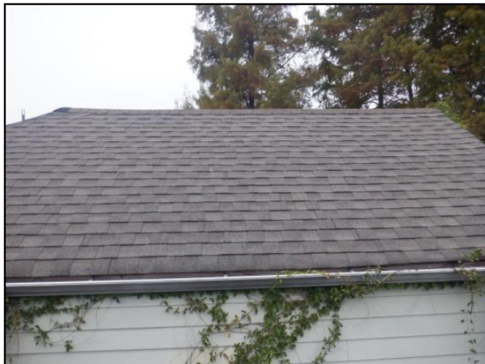
General View of the Roof System
