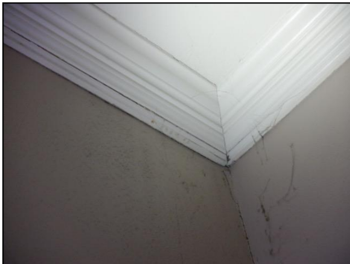
Water damage
