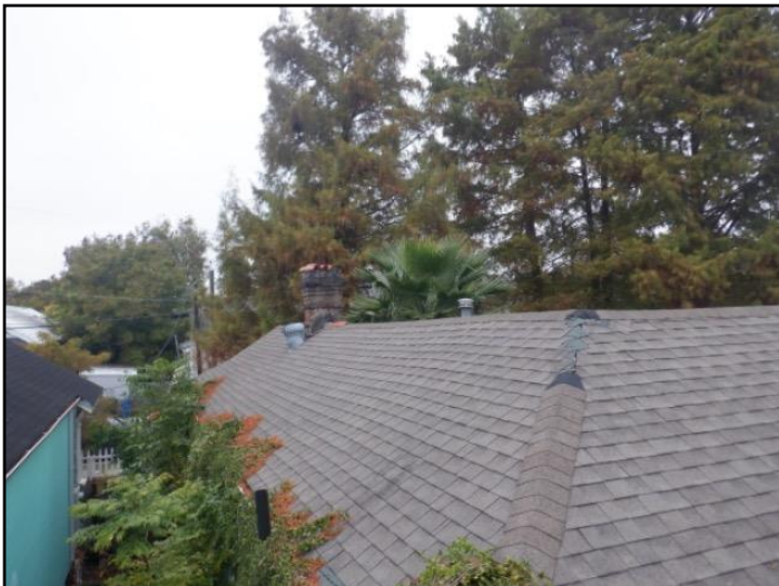
General View of the Roof System
