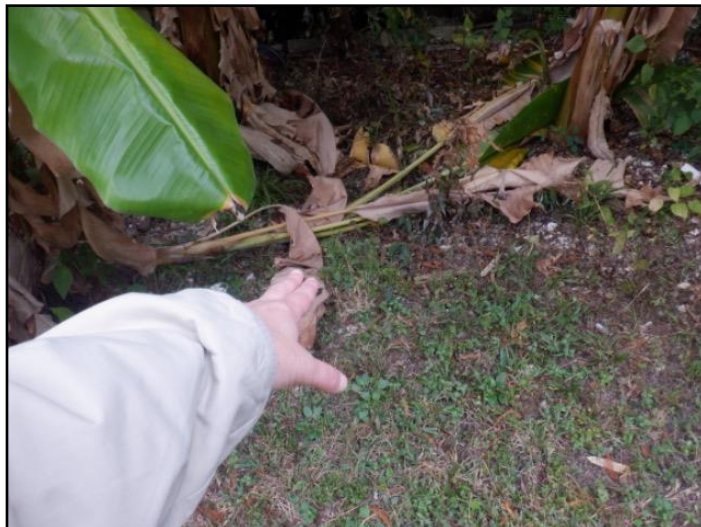
Improper slope or drainage
