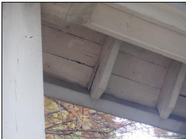
Rot/insect damage
