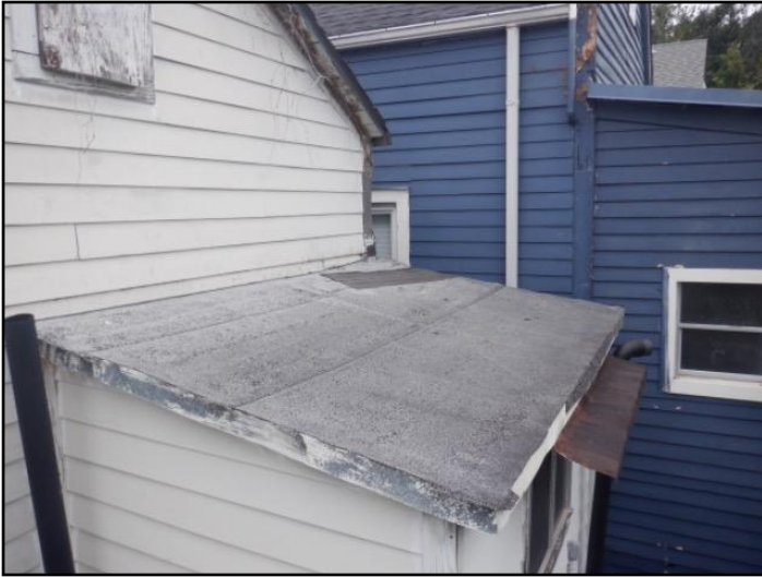
General View of the Roof System
