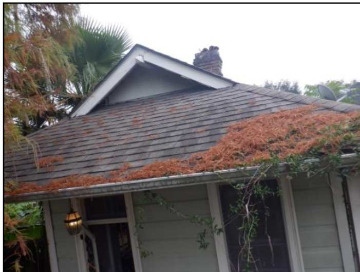
General View of the Roof System
