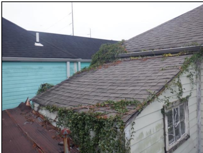
General View of the Roof System
