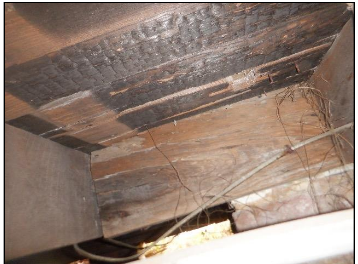
Rot and/or insect damage
