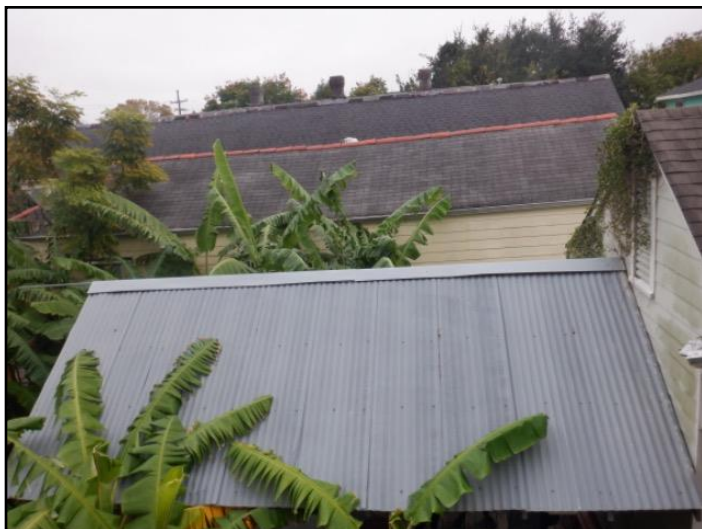
General View of the Roof System
