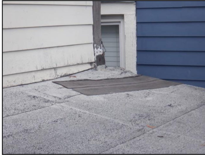
Missing flashing
