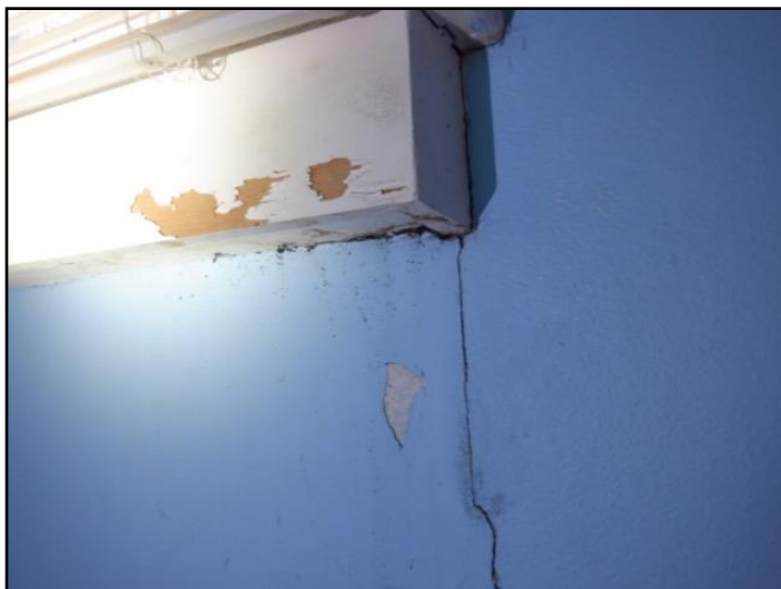
Water damage
